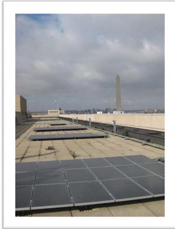
**Figure 7. Four Technology Showcase 1 kWp PV Arrays**
