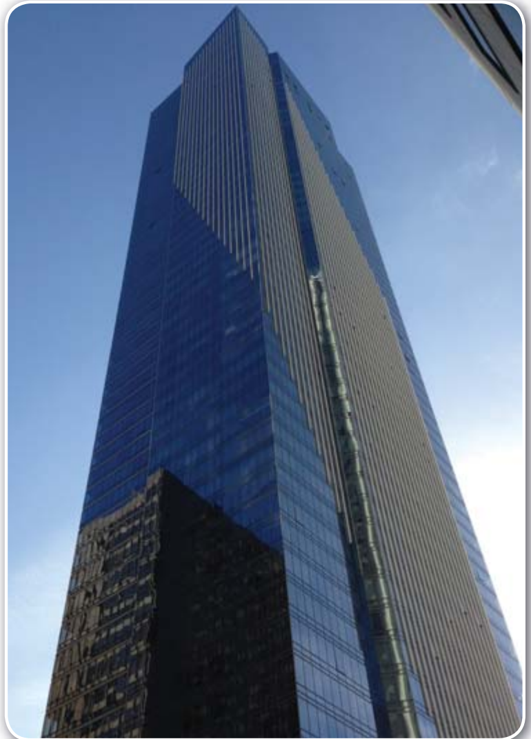
Millennium Tower in San Francisco installed PEV chargers for their tenants. See Appendix D in the Plug-in Electric Vehicle Charging Infrastructure Guidelines for Multi-unit Dwellings to read this and other case studies for MuD charger installations.
