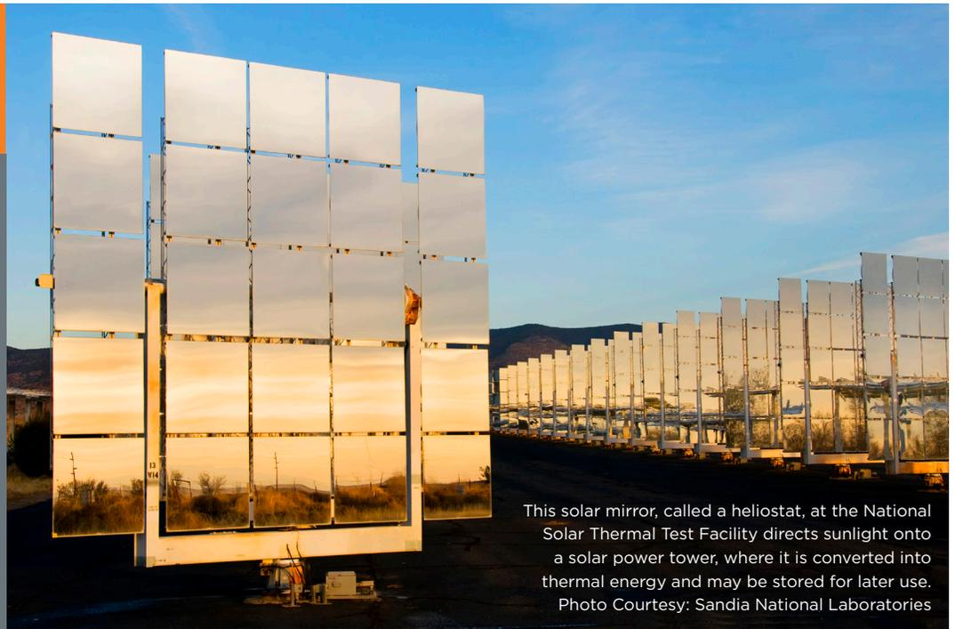
This solar mirror, called a heliostat, at the National Solar Thermal Test Facility directs sunlight onto a solar power tower, where it is converted into thermal energy and may be stored for later use. Photo Courtesy: Sandia National Laboratories
