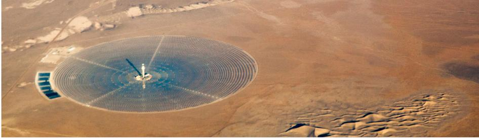
The Tonopah CSP plant is nearing completion and will be the largest molten-salt power tower CSP plant in the world, located in Tonopah, Nevada. This plant will have 8 hours of thermal energy storage, allowing it to continue to deliver power to the grid well into the night.
