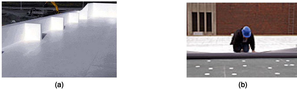
Figure 17. Reflective roof coating (a), and reflective roof membrane (b).
