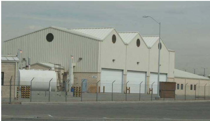
Figure 15. TEMF building at Fort Bliss with a reflective white metal roof.
